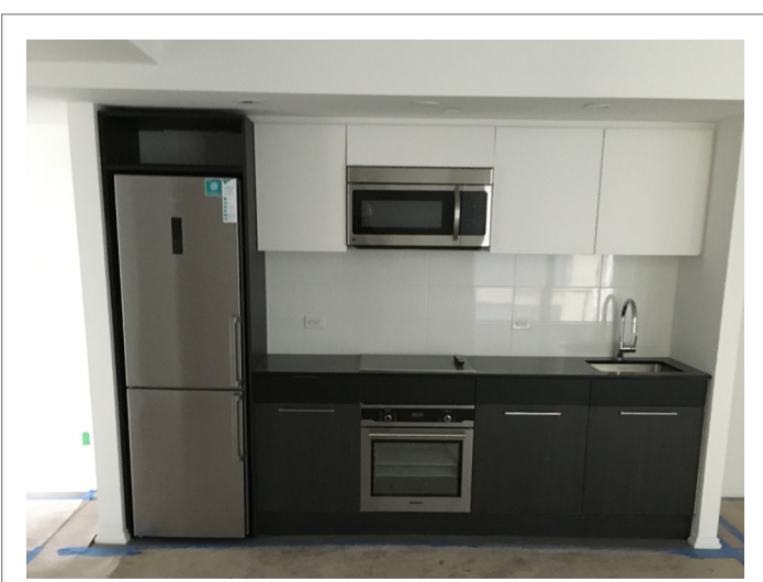
APRIL 2016 INSTALLATION OF KITCHEN CABINETRY ON THE 4TH FLOOR
