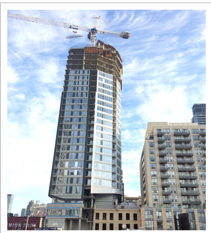
JULY 2016 WINDOW INSTALLATION UP TO LEVEL 20
