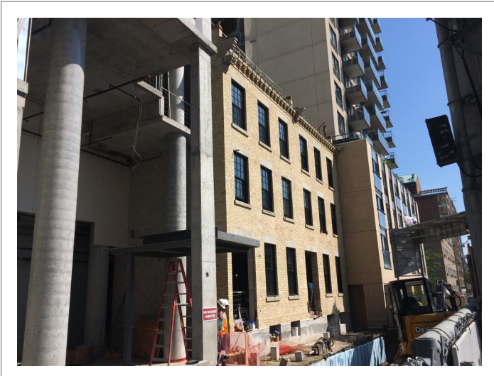
SEPTEMBER 2016 PROGRESS ON THE CONSTRUCTION OF THE HERITAGE HOUSE
